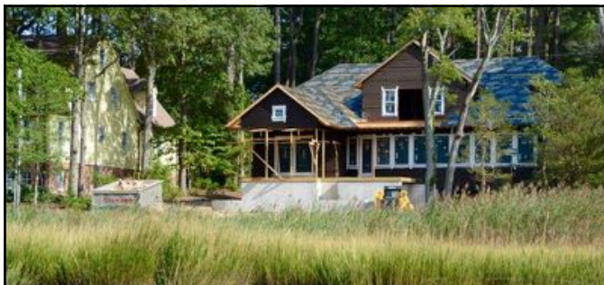
Zoning and land use ordinances in certain areas require more extensive buffer zones. The undisturbed vegetation zone runs from 30 to 50 feet from the water's edge, depending upon the location and nature of the waterway.
